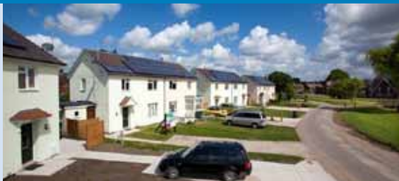
Petersfield – the rehabilitated houses showing solar panels
