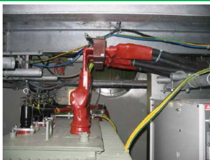
Fig. 4 Current transformers installed at transformer
